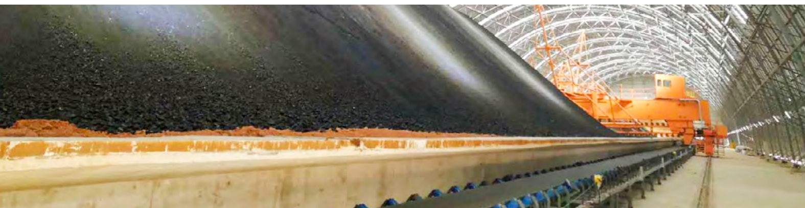
© Cleaning Line of Qilianshan Cement Co., Ltd.
