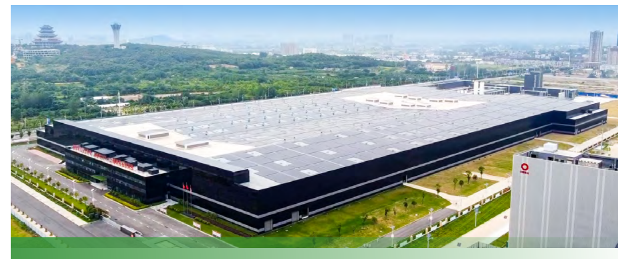
④ Triumph Science & Technology's Stand-alone 10MW Thin-film BIPV Application Demonstration Project
