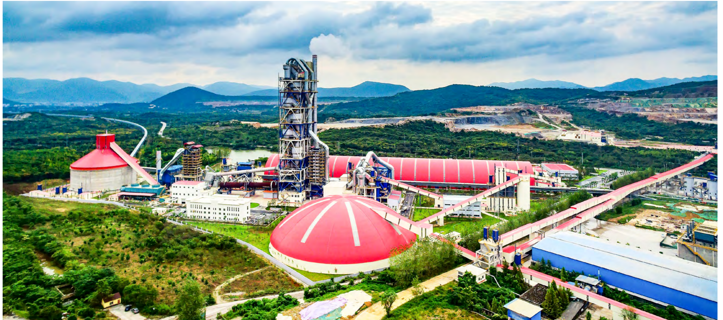
© A Panorama of Huaikan South Cement Company Limited
