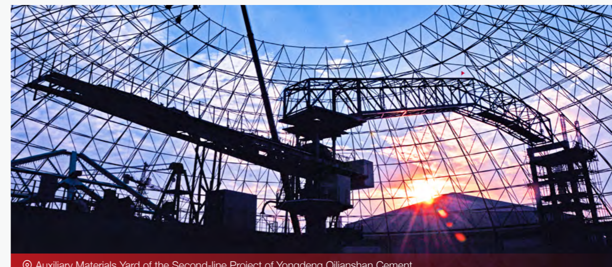
Auxiliary Materials Yard of the Second-line Project of Yongdeng Qilianshan Cement
